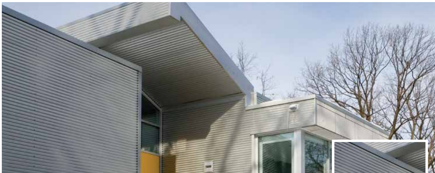
Science Addition and Allied Health Expansion, Glen Oaks Community College, Centreville, MI, USA
