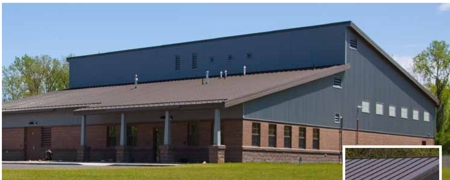
Allegan Water Treatment Plant, Allegan MI, USA
